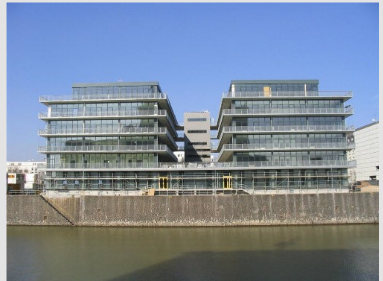
DE-CIX Competence Center @ Kontorhaus Building Frankfurt Osthafen (Docklands)
